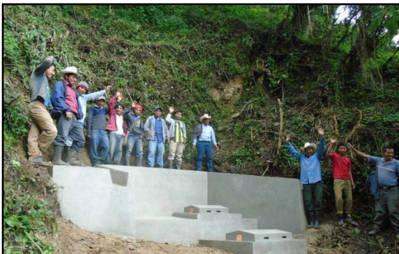
Construction of cement spring capture for the water system in Granadillas community.
