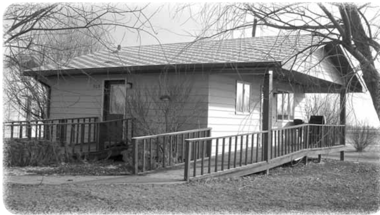
The Bismarck North Star and Bismarck Prairie Rose Lions Clubs jointly adopted Apartment 925, one of two cabins at the Great Plains Assistance Dogs Foundation facility near Jud, for renovations this past March.
