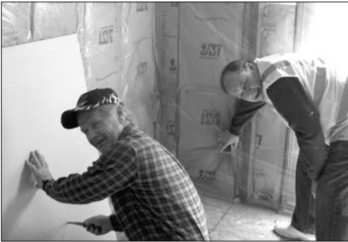
Steve Johnson and Bob Everson (Davenport Lions) installing drywall.
