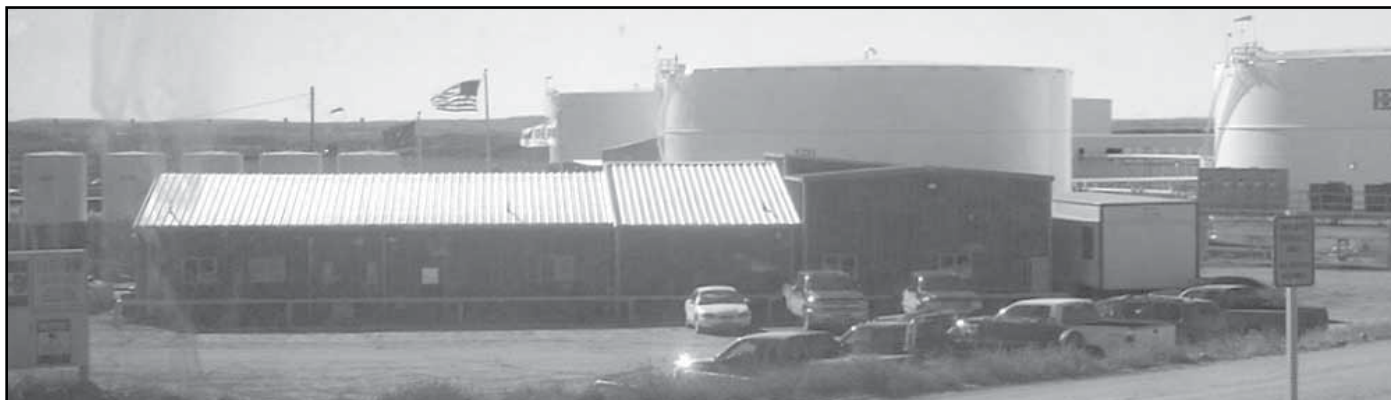
The first stop on the four-hour Bakken Oil Field Tour was at the Bakken Oil Express (BOE) depot, a unit train loading facility three miles west of Dickinson.
