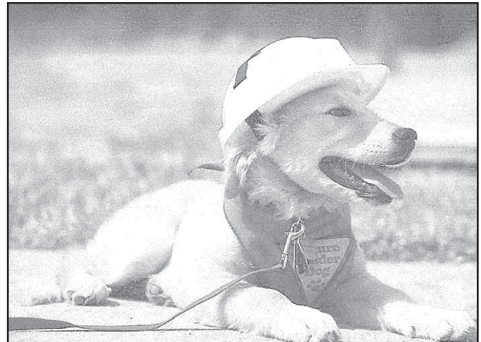
A future Leader Dog is happily supervising the early construction phase of the Leader Dogs for the Blind kennel building project.
