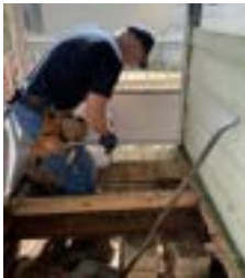
Nick removing old deck
