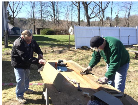
Left: Don Scott and Bill Henson scrape years of rust off of heating enclosures before applying fresh paint.
