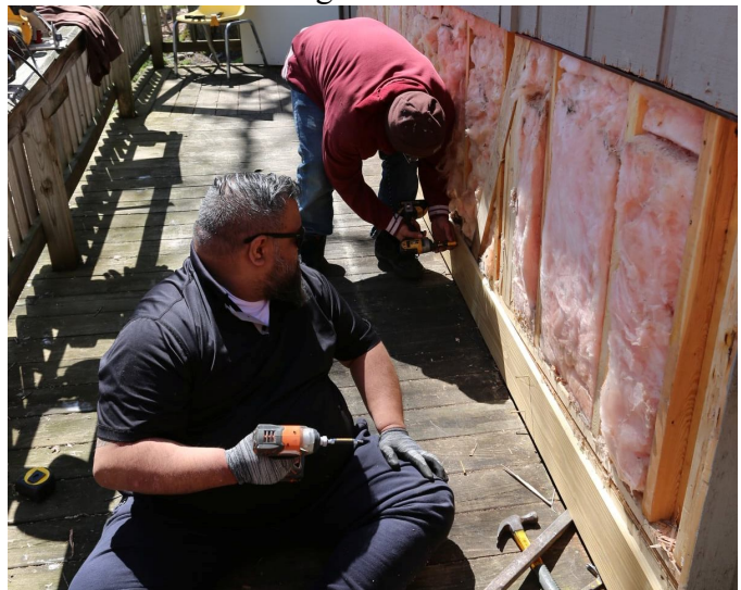
Replacing siding boards on cabins
