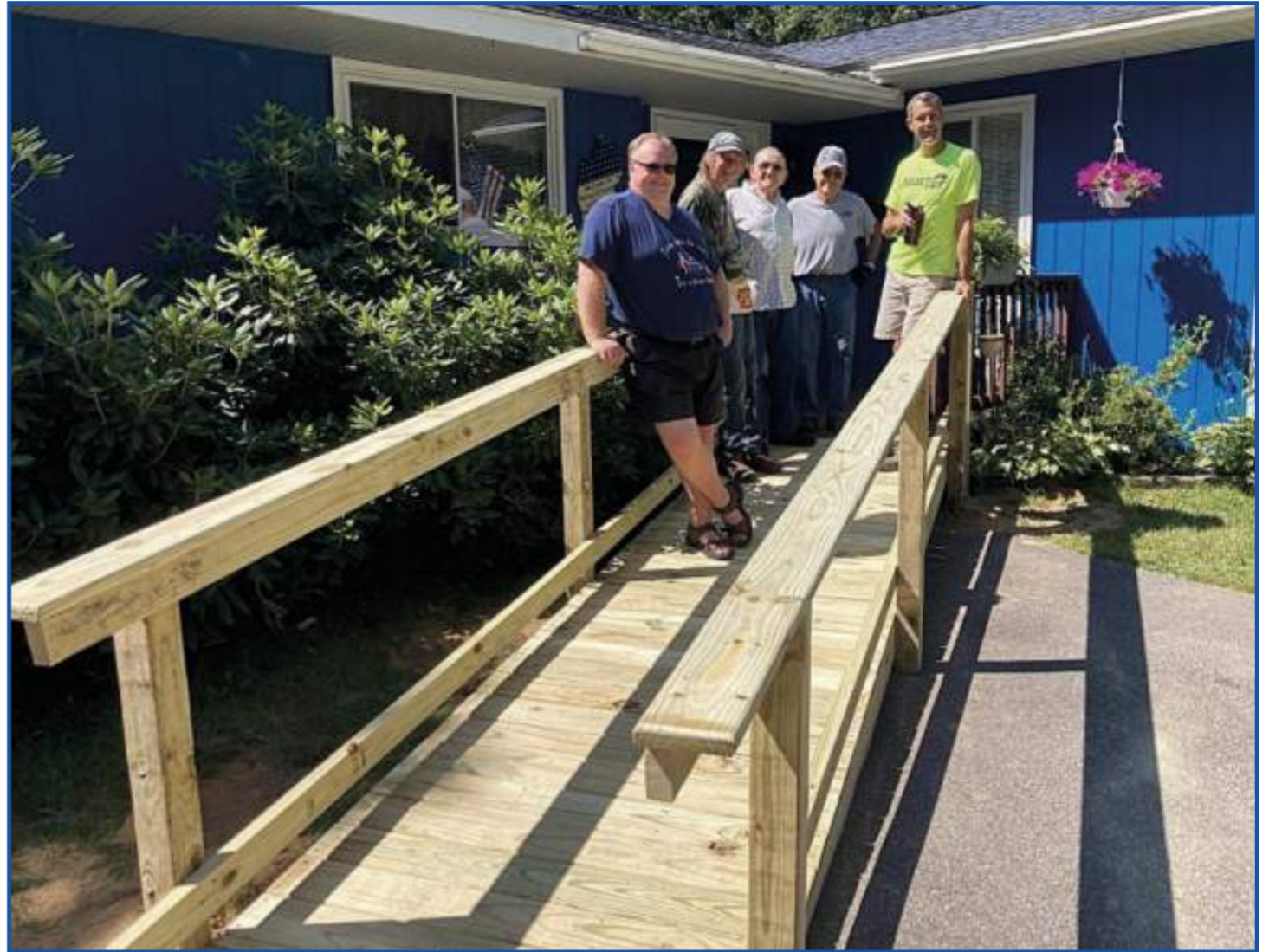
Picture Ramp104: Scott Busich, Rick Stanley. Homeowner, John Novak, Tony Priebe
