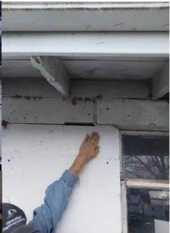
Various pictures of the damage to the Oakland City Lions Club House. The roof was lifted up and slammed down cracking the block wall.
