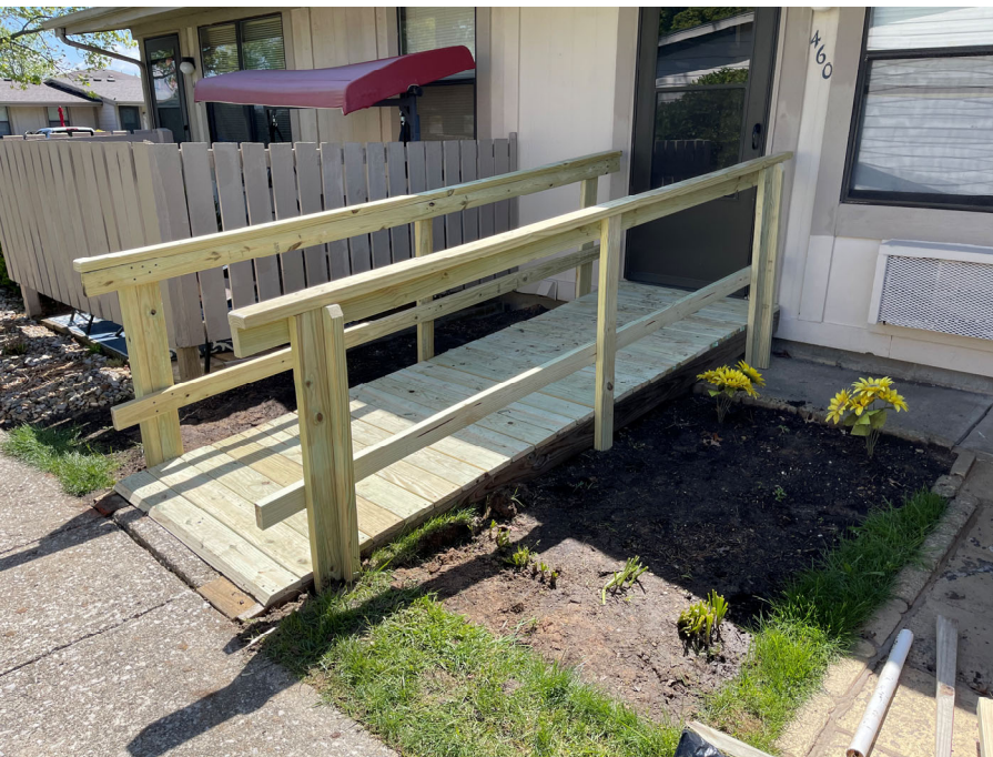
Left: Photo shows a new 12 ft ramp built at Ridgeview Apartments
