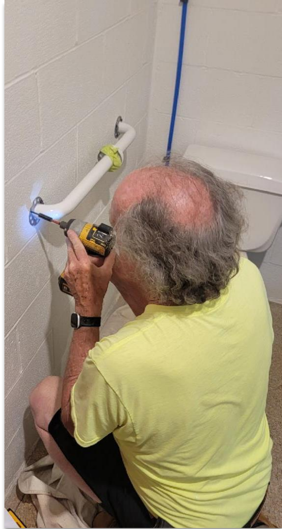
Lion Dennis McAvoy installing a grab bar in the restroom
