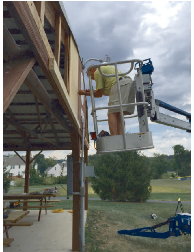
The Dillsburg Lions Club repaired its pavilion at Logan Park and replaced its timeworn signs on the pavilion. Lion John Cocklin works on installing new T-111 siding on the pavilion.
