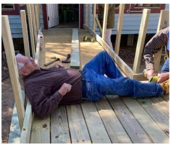
**Above:** While one PDG steadies a key corner post another tests the strength and integrity of the ramp structure. Everyone works during a ramp build.
