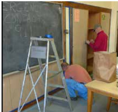
Lions Fred Kellett and Nick Daddario taping the wood that is not to be painted.
