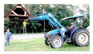
The photos show Lion Dan on the tractor operating the fork to lift the roof section up 10' and settle it on the posts with Lions Duane and Jim coaxing it into place and securing it.
