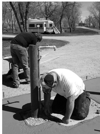
Lions Dustin and Morgan putting final touches on new sani station.
