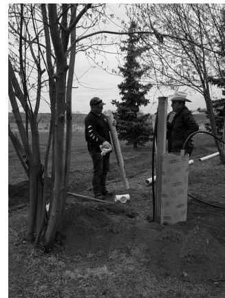
Discussion concerning laying pipes in the campground
